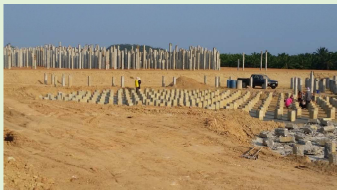
Tank Farm Construction
